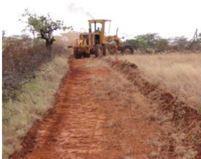
Fire break construction(use of heavy machinery
