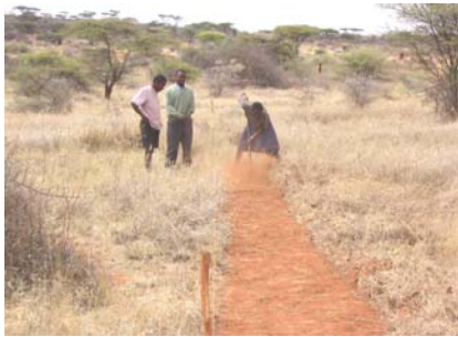
Fire break construction Manually)
